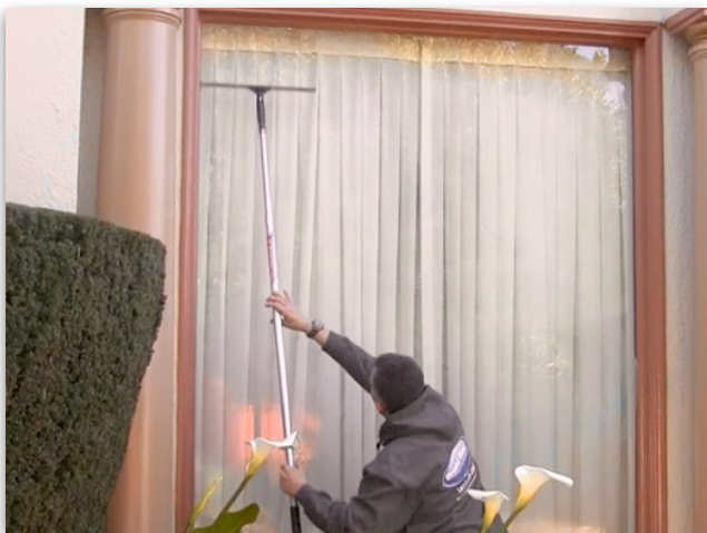
After cleaning the entire window surface with a wet sponge, use a squeegee to dry it.
